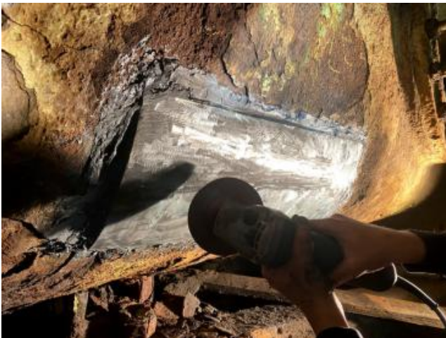
(Fig 3) - Steel Plate bonded with Industrial Metal over the repair area.
