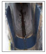
Extremely wet conditions and water leakage/flow required a strong polymer that would bond to wet/underwater conditions. Sealrite WBC used for repairs of cracked trenches for holding tank.
